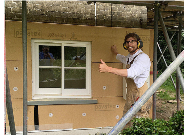
Regenerative Trait: Upskilling local community Mike's Cottage, Pamphilon Architects
